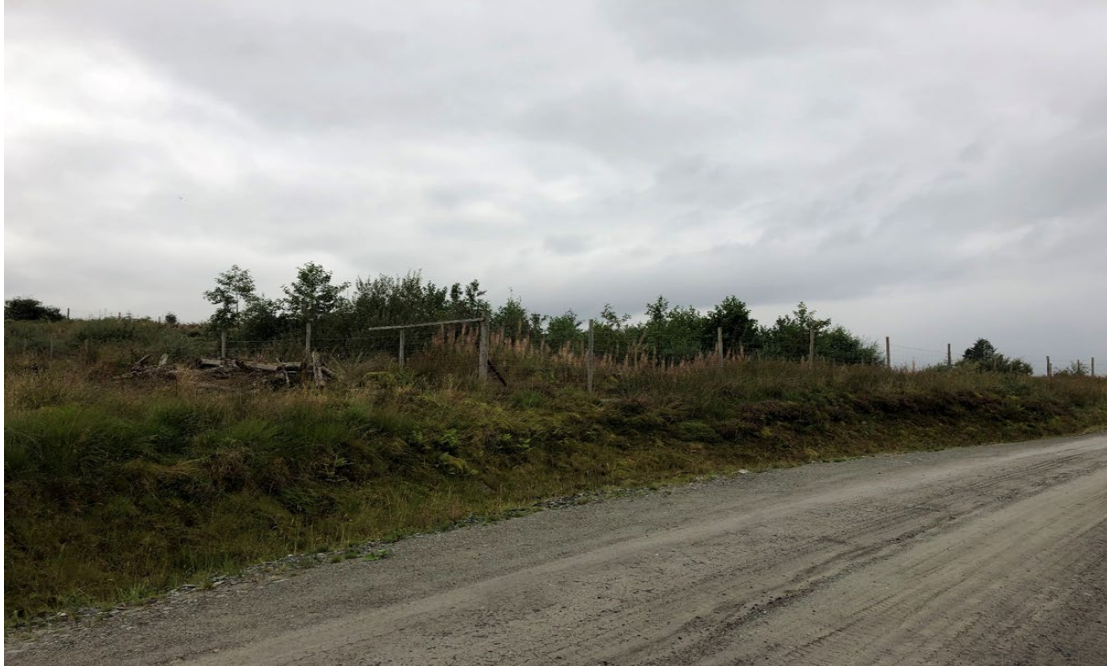
Plate 5.1: Looking west to tower 25.
